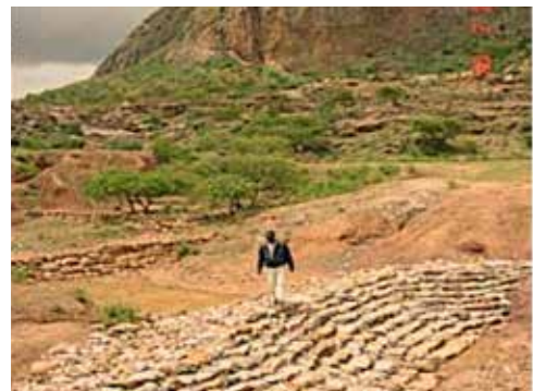
Figure 22. Wedge-shaped loose-stone check dams are particularly effective for erosion control
