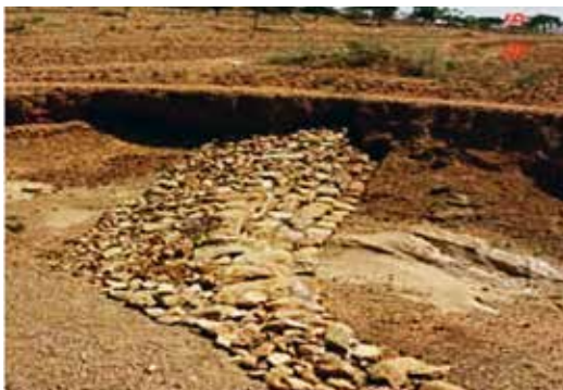
Figure 22. Wedge-shaped loose-stone check dams are particularly effective for erosion control
