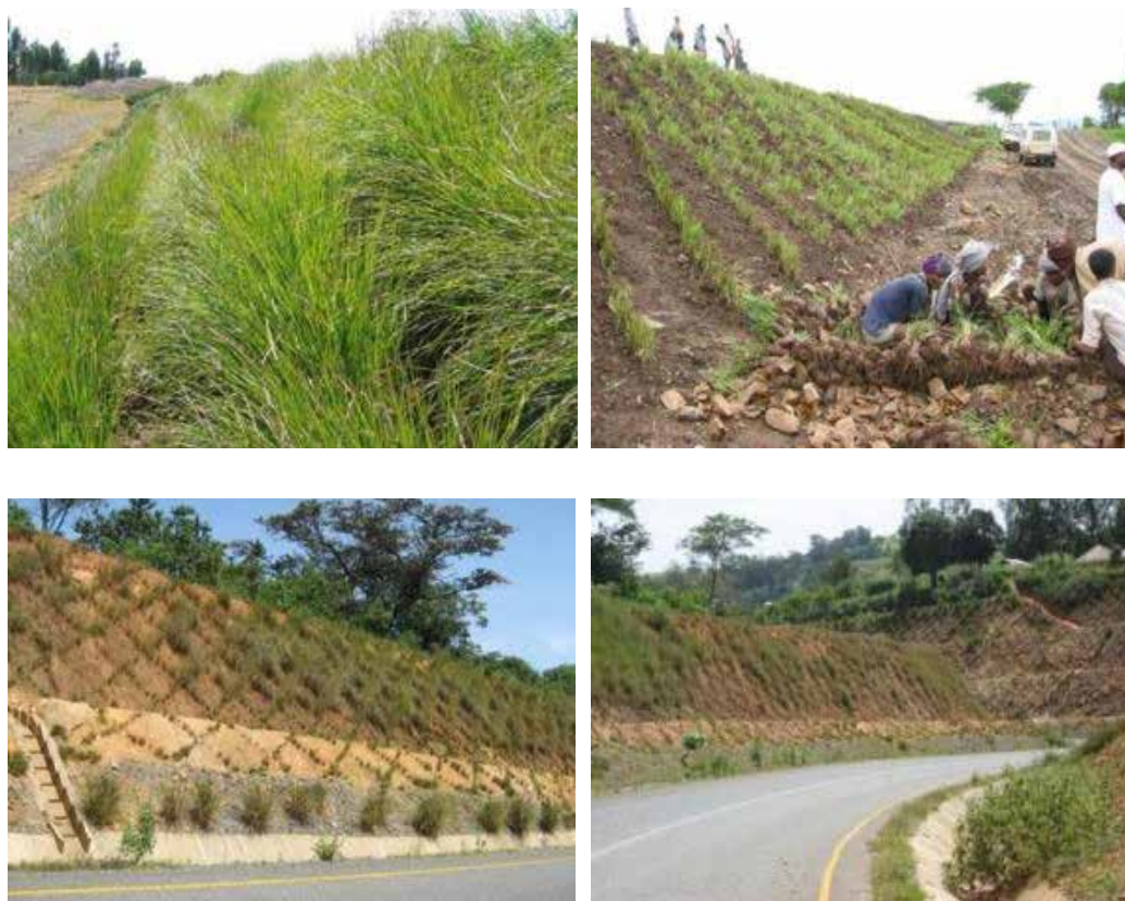
Figure 44. Bio-physical stabilisation of roadsides on the Bahir Dar–Gonder road (upper) and Assosa–Nekemte road (lower)
