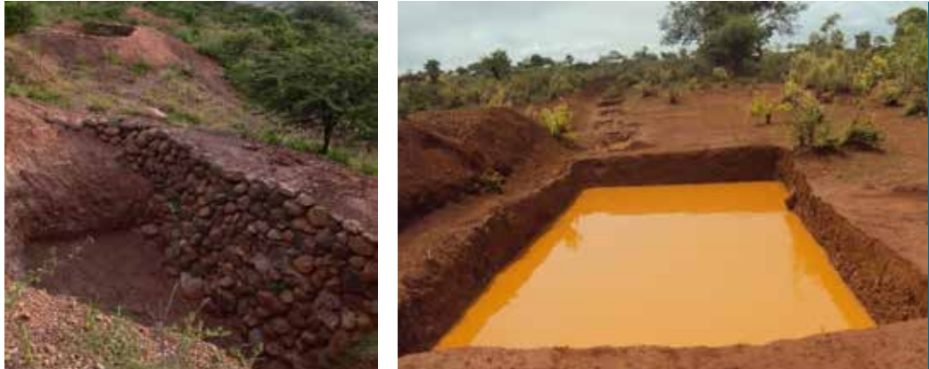
Figure 33. Percolation ponds constructed on communal land
