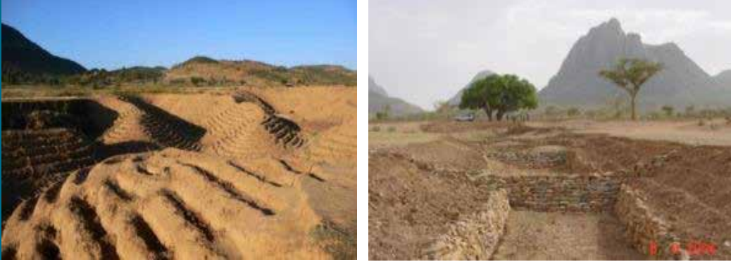
Figure 26. Reshaping gully walls is labour intensive and consumes arable land but does increase stability
