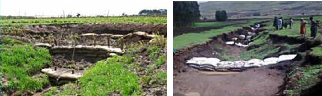
Figure 23. Sandbag check dams
